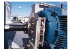
The Addax Cooling Tower Brake is a mechanical, manually-actuated caliper disc brake for stopping, holding and locking out cooling tower fans. It easily adapts to the motor hub of the Addax Composite Coupling.
